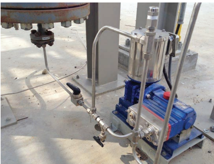
A P200 replaced a conventional single diaphragm pump in a refinery application to eliminate pulsing flow and noise.
